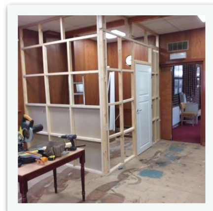
Accessible toilet being formed.
